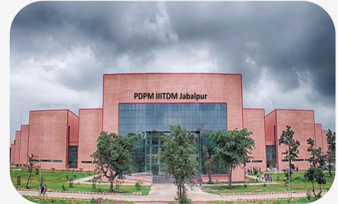
Electronics and ICT Academy, Phase II
