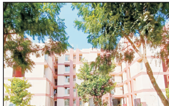
Nagarjuna Hostel (PG Married Accommodation-Phase I)
