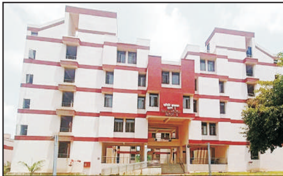
Panini Hostel (PG Bachelor Accommodation-Phase II, Block A)
