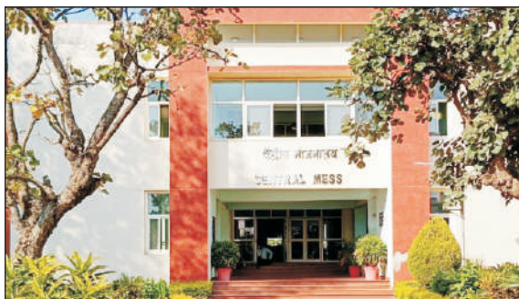
Central Mess (Mess and Dining Hall)
